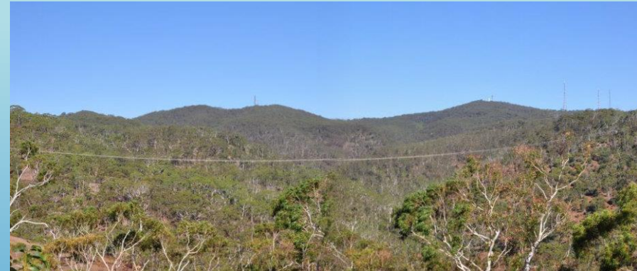
With transmission wires 5.92
